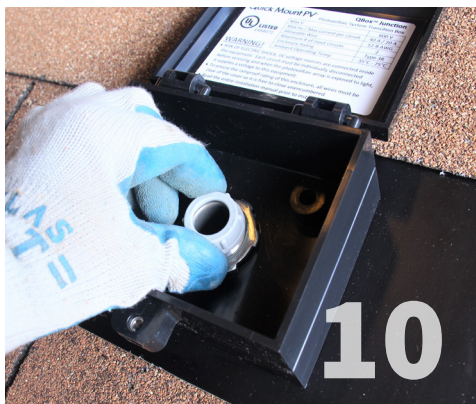
Finish Conduit Attach: Hand tighten threaded conduit cap to secure conduit nipple in place. This will hold the QBox flashing in place when securing it to the roof.
