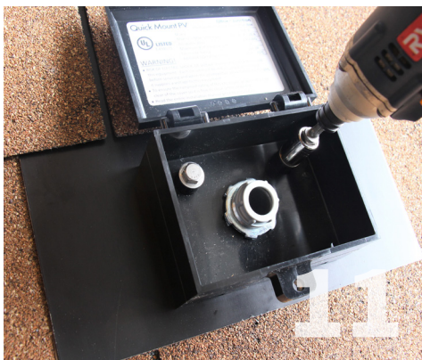
Secure to Roof: Screw the anchor bolts with sealing washers through the mounting holes and into the roof sheathing securing the QBox to the roof. No pilot hole is required.
