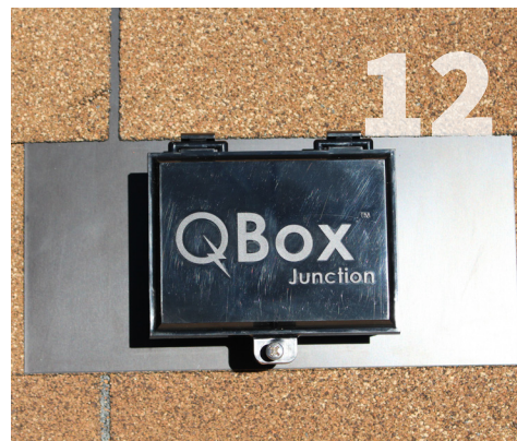
Close Lid: Close and thread the bolt into the nut by hand. Then using a #3 Philips drive, turn bolt until the top and bottom tabs securing the bolt are flush.
